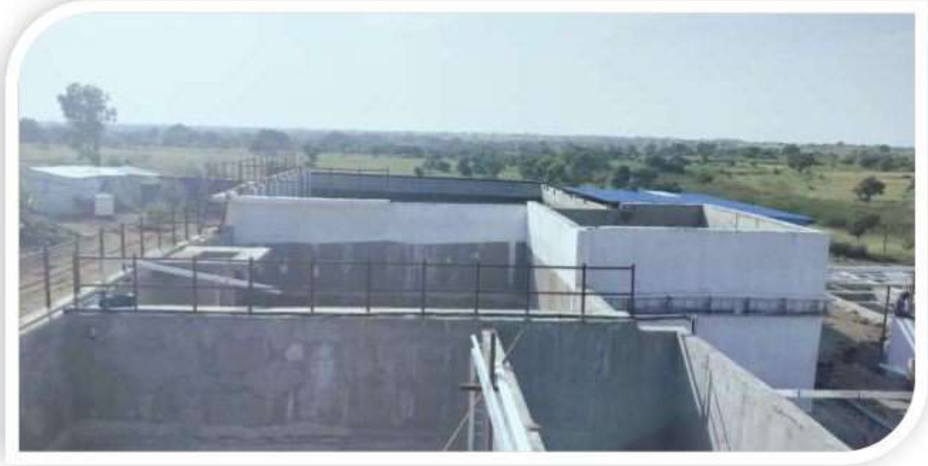
Photograph: Under construction CPU
