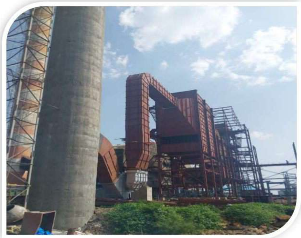
Photograph: APCE- Stack with ESP
