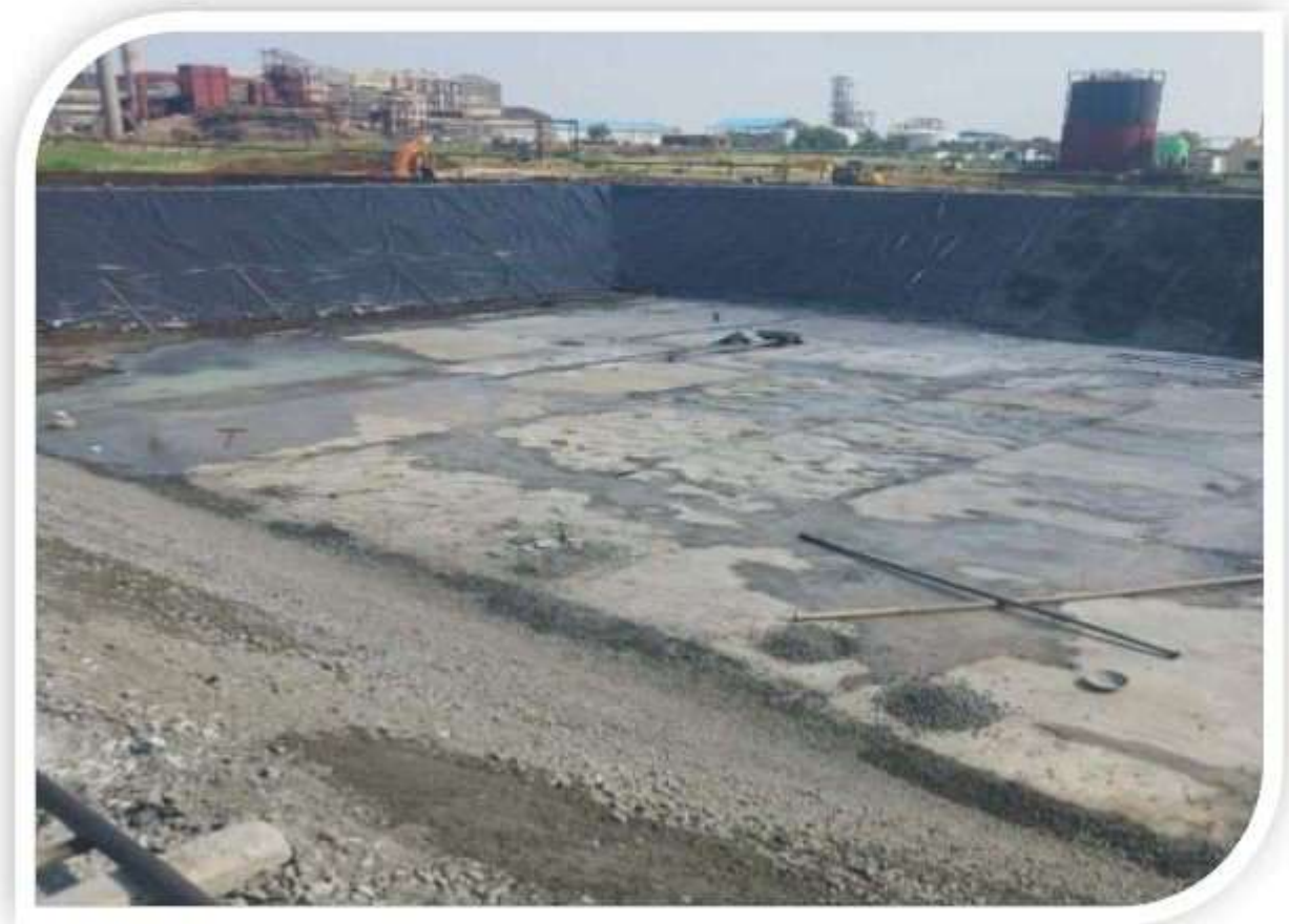
Photograph: Under construction Spentwash storage tank as per CREP guidelines
